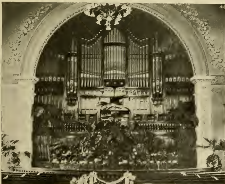
INTERIOR OF METHODIST CHURCH.
